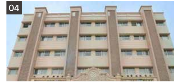
04 Hospital, Ahmedabad ( 357 HP )
